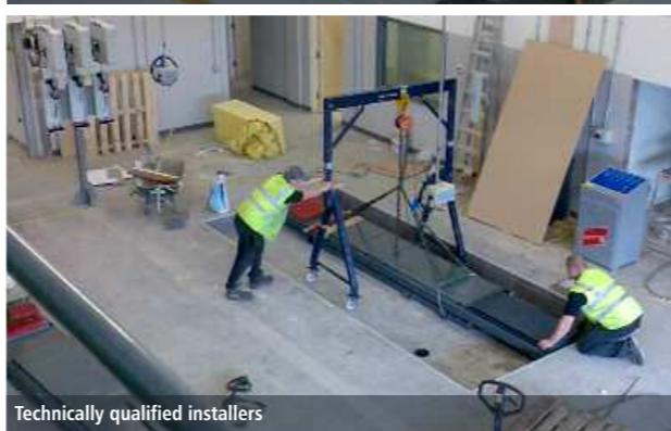
Complete qualified services installation
