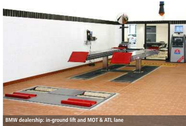
BMW dealership: in-ground lift and MOT & ATL lane
